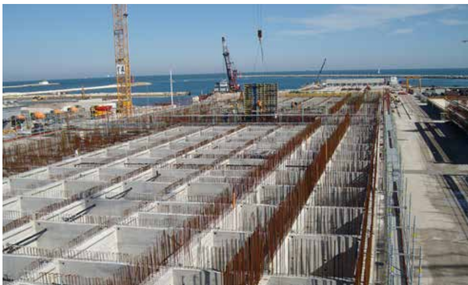
Venice Malamocco harbour pass. Construction of the structures forming the foundations of the MO.S.E. system that was conceived to protect Venice from sea-level rise. The four barriers are now completed.
